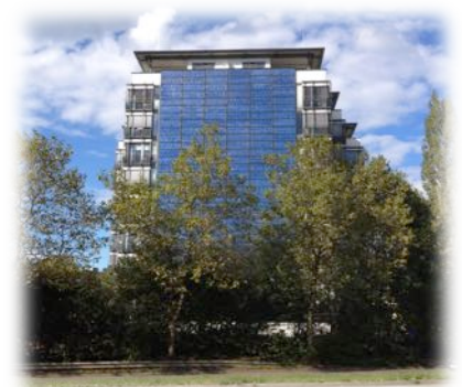
Solar high-rise on Berliner Allee
